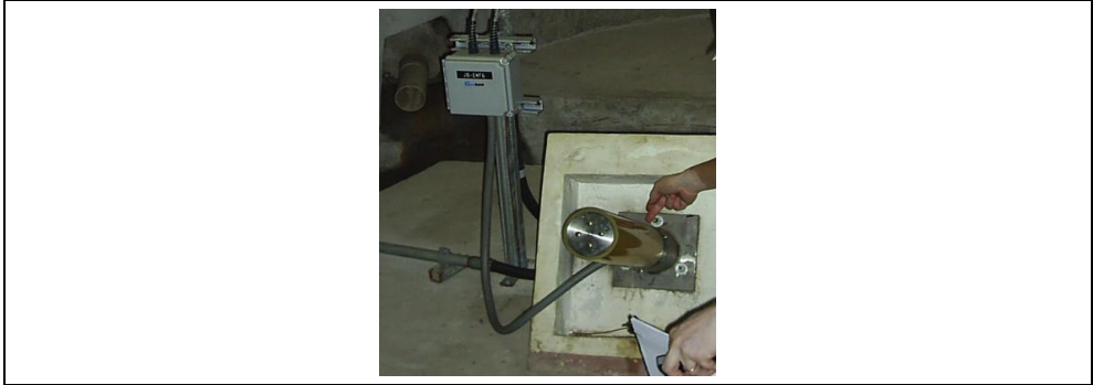
Fig. 5. Automated extensometer installed in Itaipu's rock foundation.
